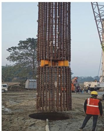
Figure 1 Bi-Directional Load Cell positioned inside the reinforcement cage
