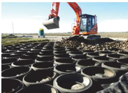
**Figure 8** Placement of tyre cells in a field project
