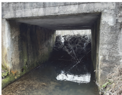
Figure 14 Water duct buried
