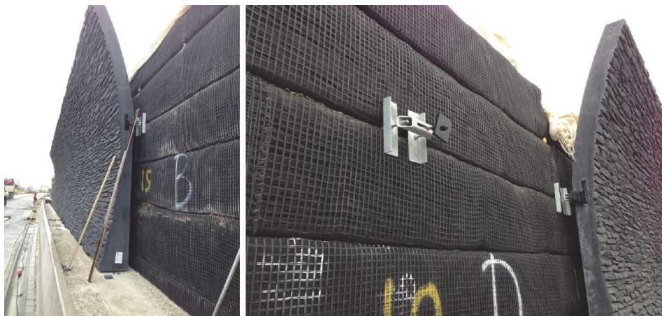
Figure 5 Full height concrete panels installed as a passive facing (Vrijenburgweg, Netherlands)
