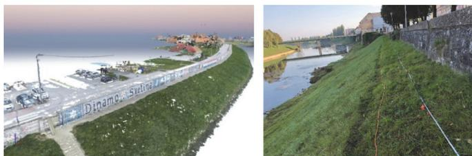
Figure 2 A 3D point cloud of riverbank (left) and geophysical investigations (right)
