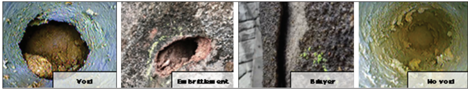
Figure 5 Conditions identified in core sampling
