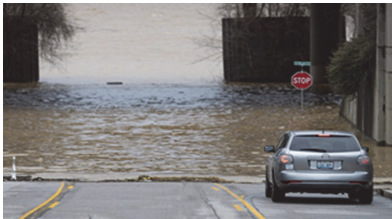
Figure 3 Consequence of flooding on road infrastructure (Source: jpdcfbh.ba)
