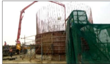
j) Concrete Pouring (on site activities)
