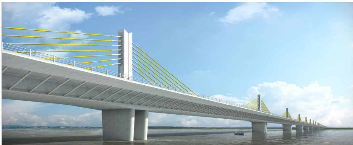
Figure 3 Aesthetic appearance of Extradosed Bridge
