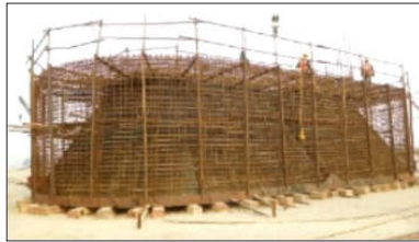
i) Rebar Arrangement (on site activities)
